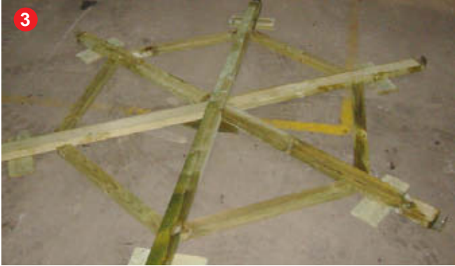
Add floor bearer separators.
