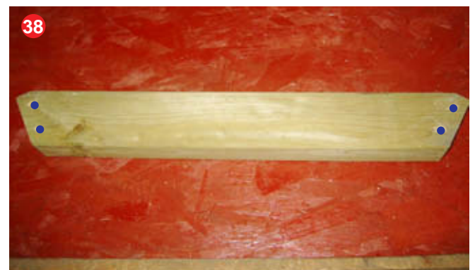
Drill 4 holes in small upright top frames.
