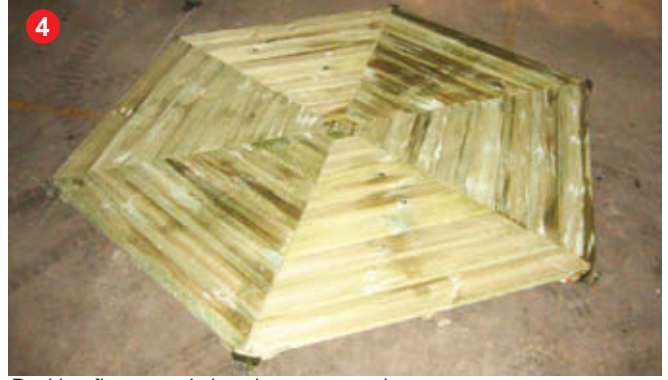
Position floor panels but do not screw down.
