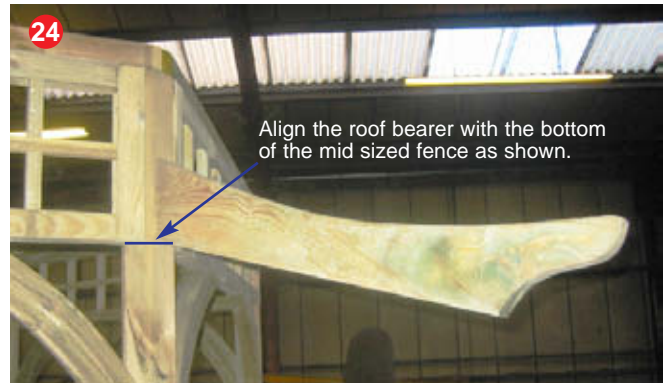
24 Align the roof bearer with the bottom of the mid sized fence as shown. Screw through the pre-drilled hole of the upright into the roof bearer.
