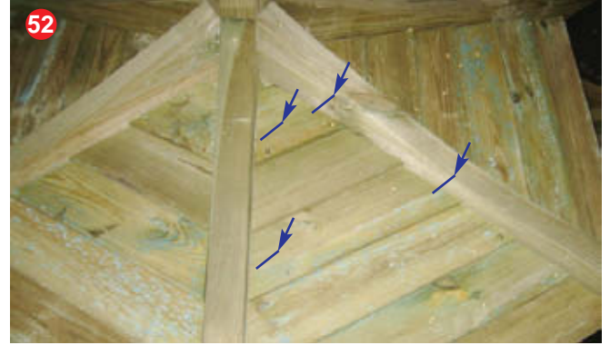
52 Secure roof panels to the top roof rafters using 4 x 50mm screws per panel.
