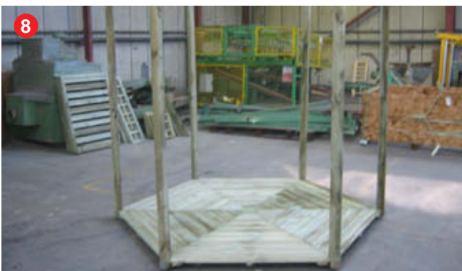
All uprights secured in place.
