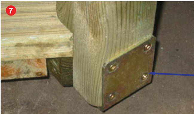
Secure uprights in place with 4 x 50mm screws.
